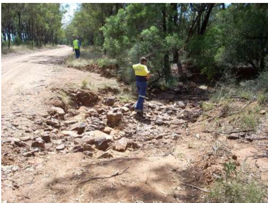
Figure 2.5 Gully draining into Pine Creek Tributary 1 (Longwall Panel 3)
